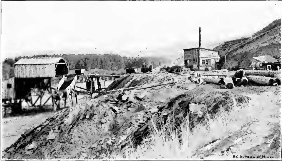
Diamond Vale Colliery—No. 3 Slope and Tipple.
